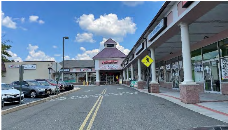
Serenity Plaza from interior driveway.
