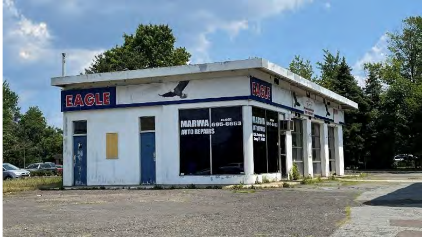
Garage and office building.
