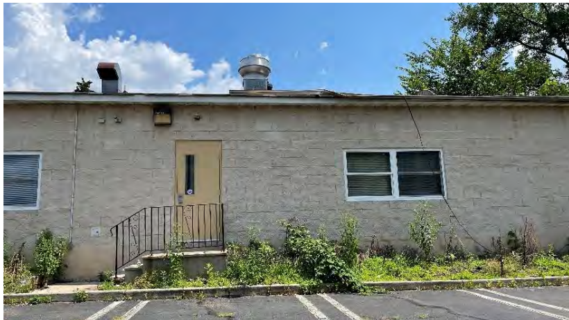
Vacant daycare rear.
