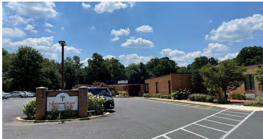
Greenwood House from Walter St
