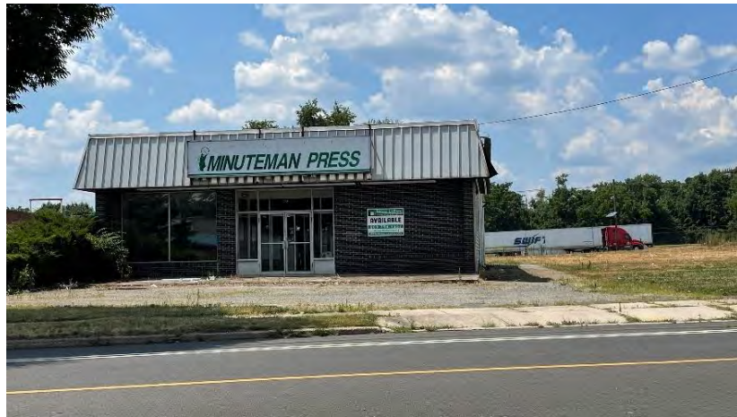
Frontage and parking lot on Scotch Road.
