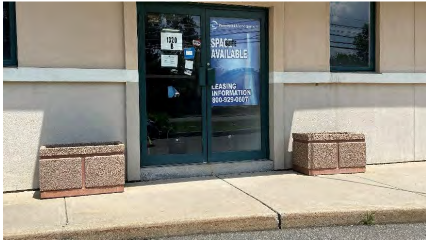
ADA non-compliant front entry on Parkway Ave.
