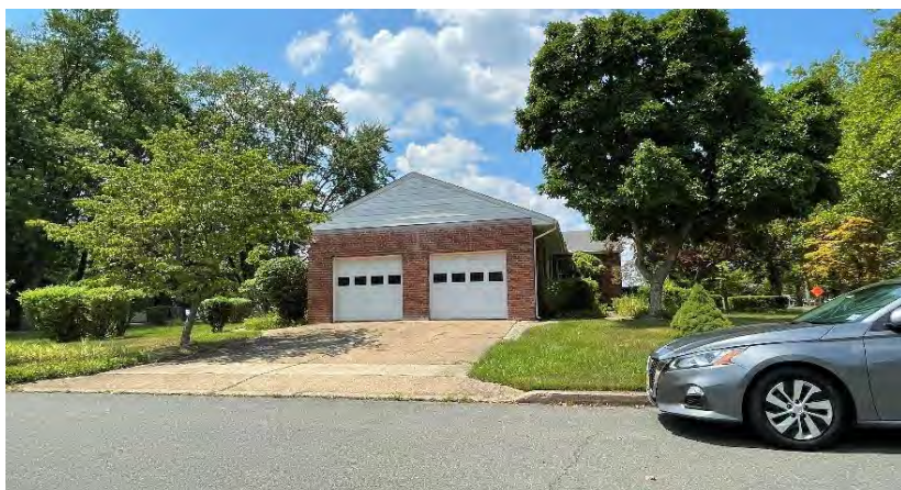
1205 Parkway Avenue from Walter Street.
