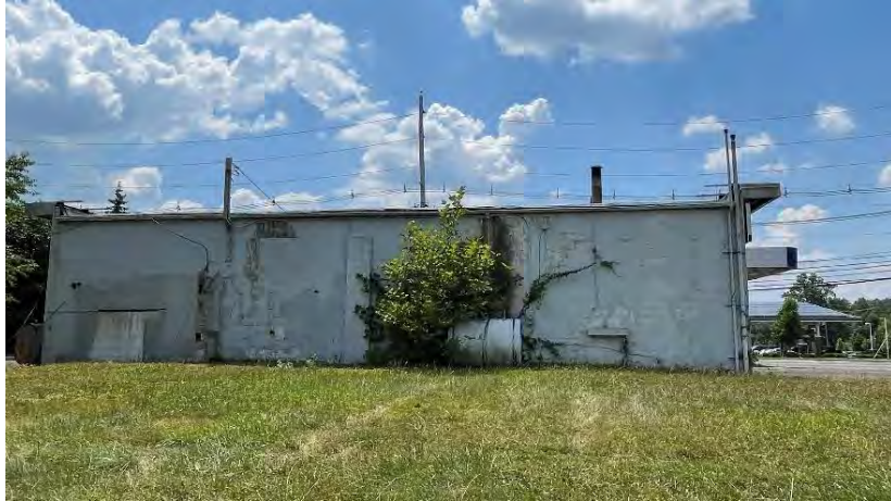
Rear façade from side yard.
