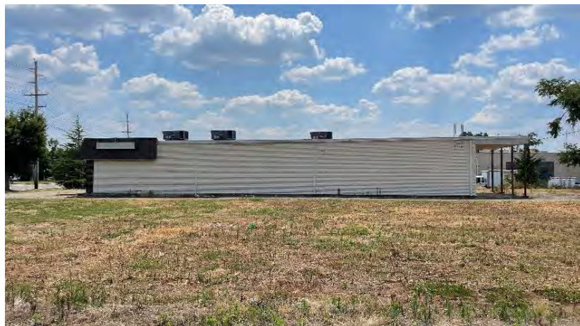
Building from unimproved side yard.
