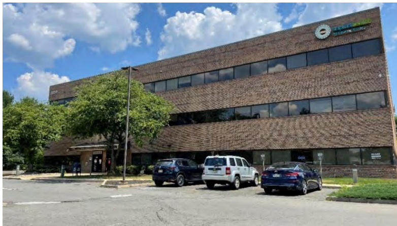
Parkway Avenue frontage.
