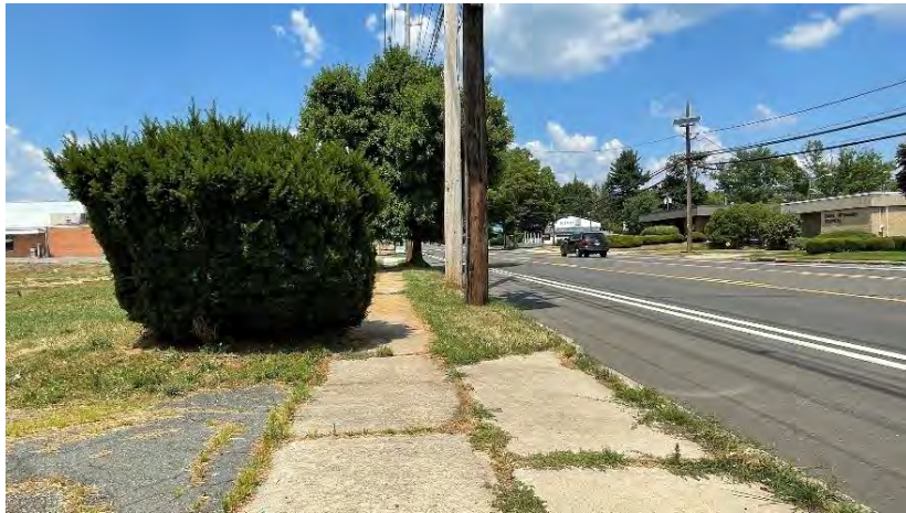
Poor visibility of oncoming traffic on Scotch Road.
